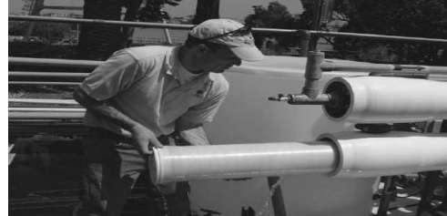
Figure 1.13 Unloading an RO membrane element from a pressure vessel [1].
