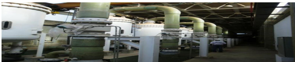
Figure 1.32 Cartridge filters
