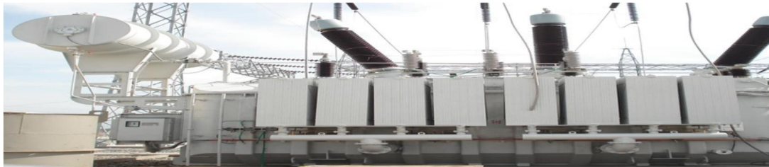
Figure 1.36 30 MVA transformer.
