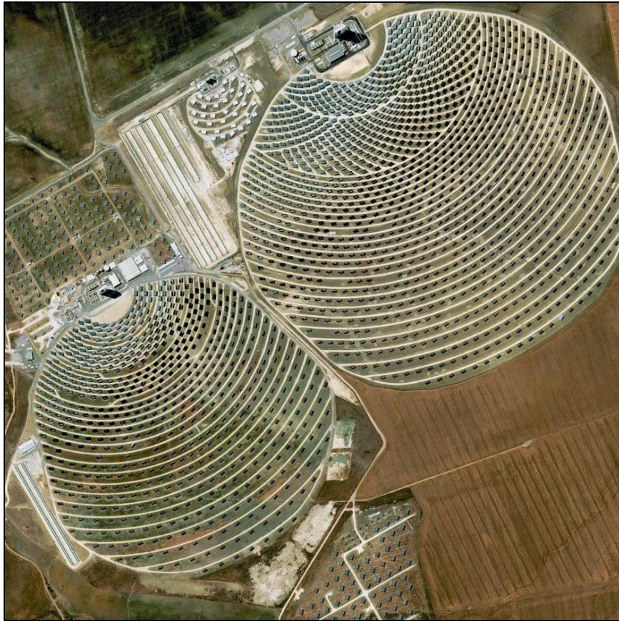
FIGURE 1.4: PS10 AND PS20 LARGE CAVITY CENTRAL RECEIVER POWER PLANT. SPAIN [16]
