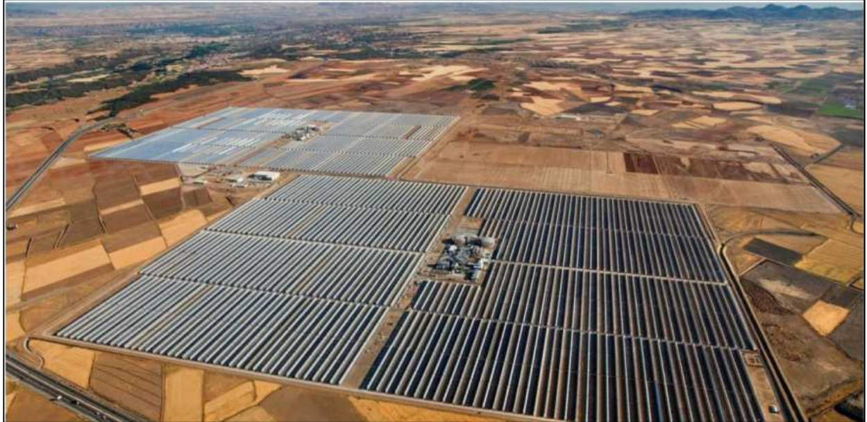
FIGURE 1.2: PARABOLIC TROUGH PLANT INSTALLATION IN SPAIN [14].
