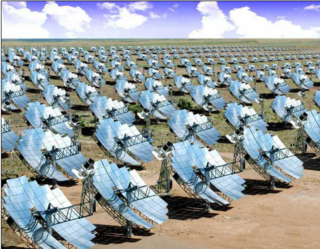
FIGURE 1.5: MODULATED DISH-STERLING POWER PLANT INSTALLATION. [17]
