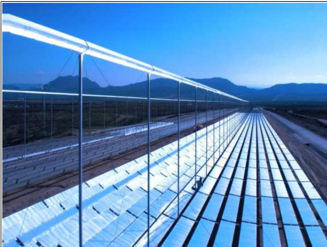
FIGURE 1.3: LINEAR FRESNEL COLLECTOR PLANT [15]
