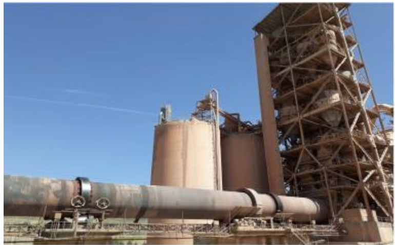
Figure 4.1-a. Pre-heater tower at the right along with rotary kiln laying in horizontal to the left.
