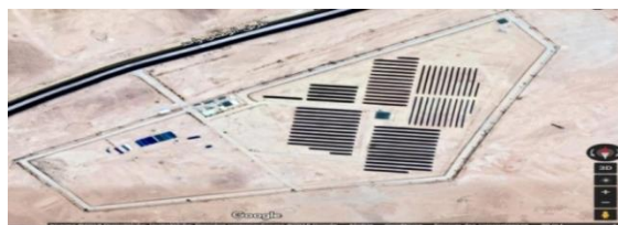
Figure 4. Satellite image of the plant of Ghardaia
