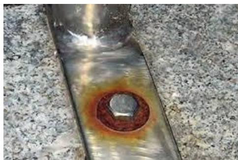
Figure I.3 : corrosion uniforme
