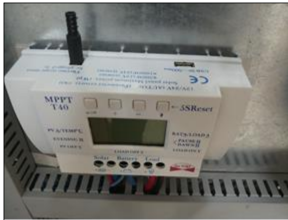
Figure 2.8: MPPT T40 Charge Controller.
