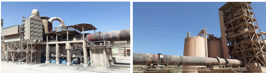
(a) cooler system with its heat exchanger and (b) pre-heater tower at the right along with rotary filter to the left and kiln end appears to the right. kiln laying in horizontal to the left.
