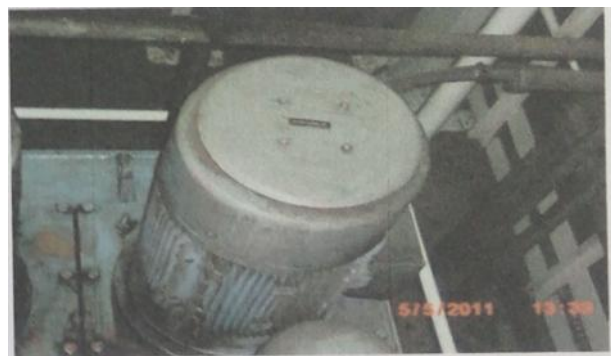
Figure III.4 Pompe principale de graissage.
