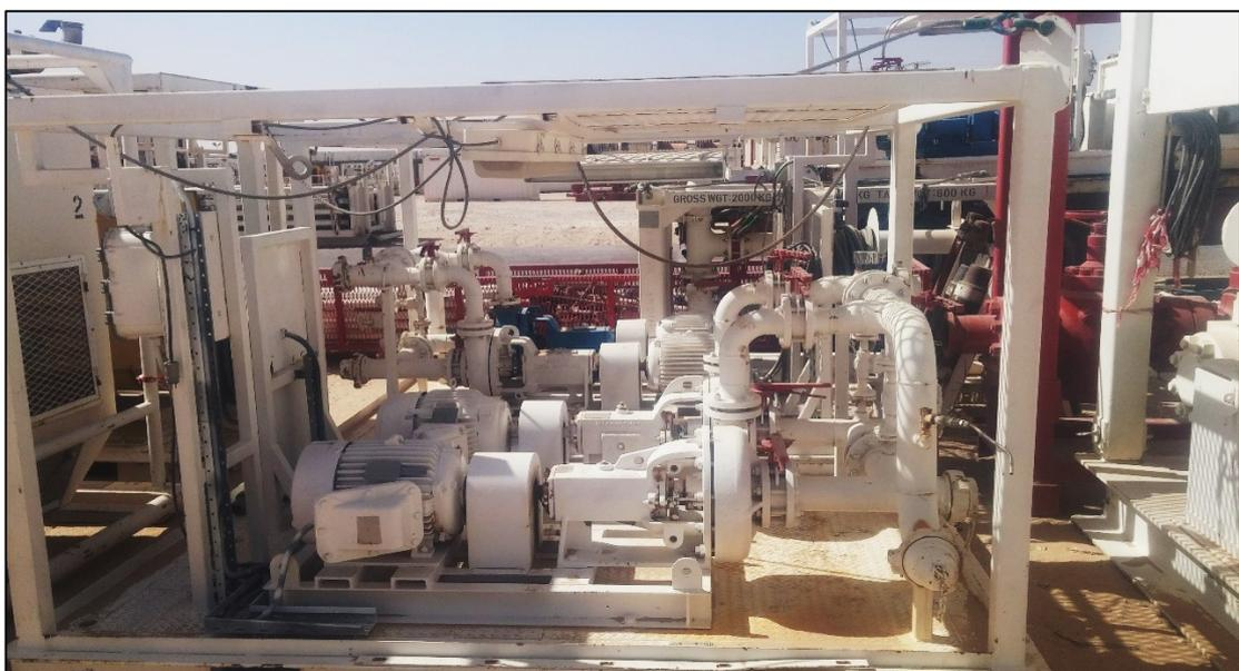
**Figure 4.11 :** Back-pressure Pump.
