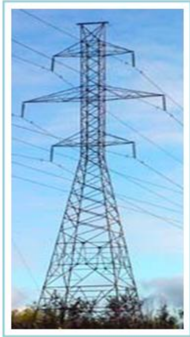
Figure (II-7): Pylône de type Nappe
