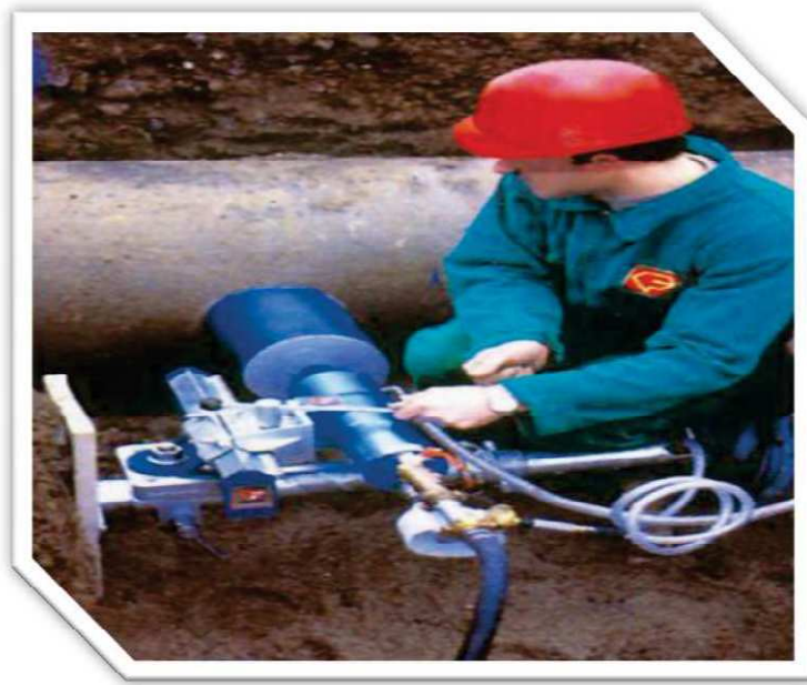
Figure 20 : Carottage horizontal.
