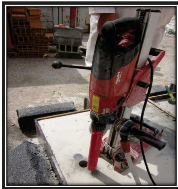
Figure 19 : carottage vertical
