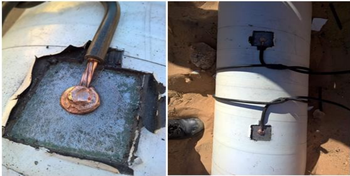
Figure III. 5 Soudage des câbles de raccordement.
